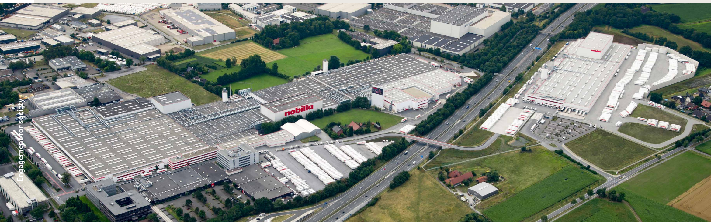
nobilia Plant I in Verl and Plant III in Gütersloh
